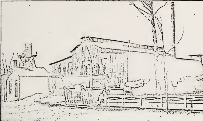
ROHM FERGUSON & SONS' MILL FROM A PHOTOGRAPH TAKEN TWENTY YEARS AGO.
